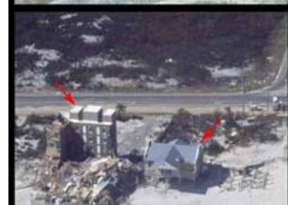
Results of a storm surge - Orange Beach, Alabama. Image by USGS
