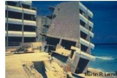
Figure 4. Eroded foundation and resulting collapse of a building on the coast following a hurricane-induced storm surge.
